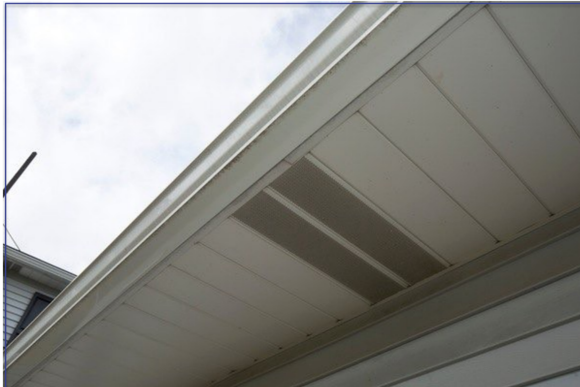
NON-HIDDEN VENT SOFFIT
