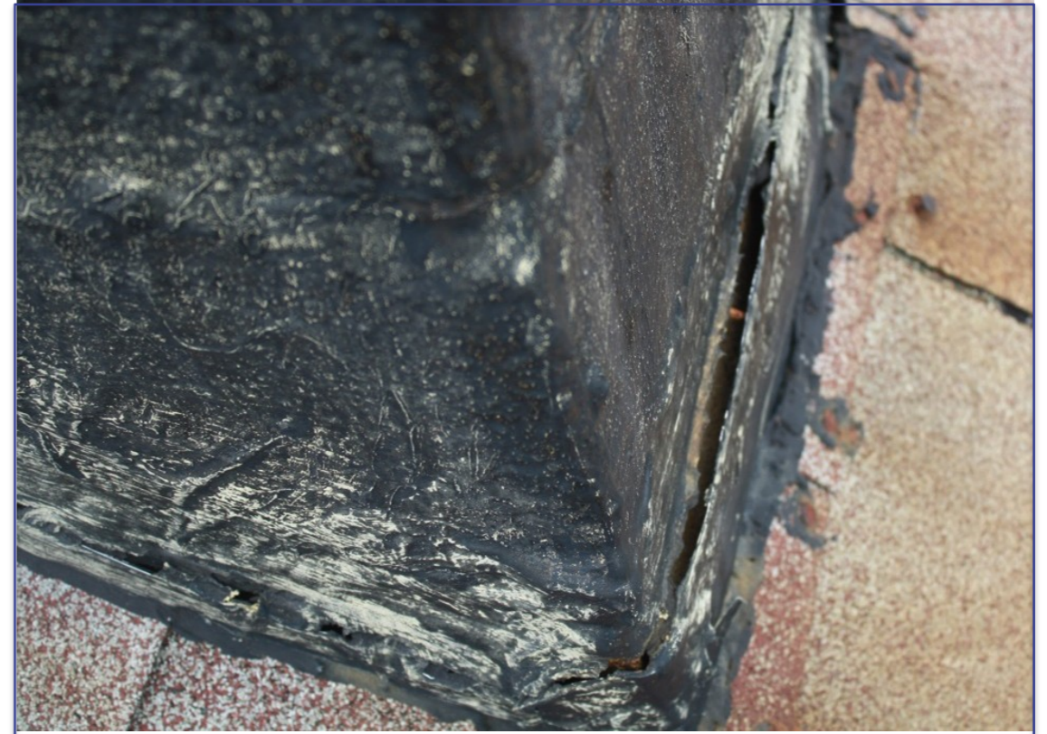
CHIMNEY FLASHING
