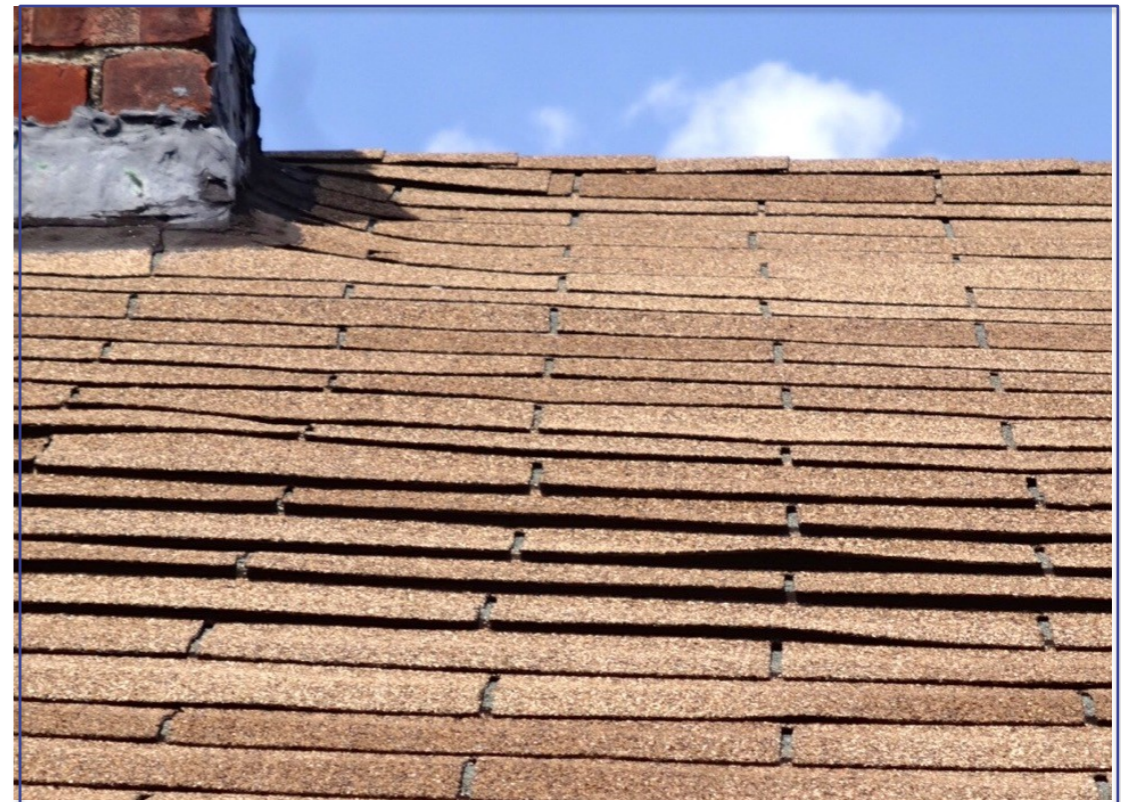
WARPED & SHRINKING SHINGLES
