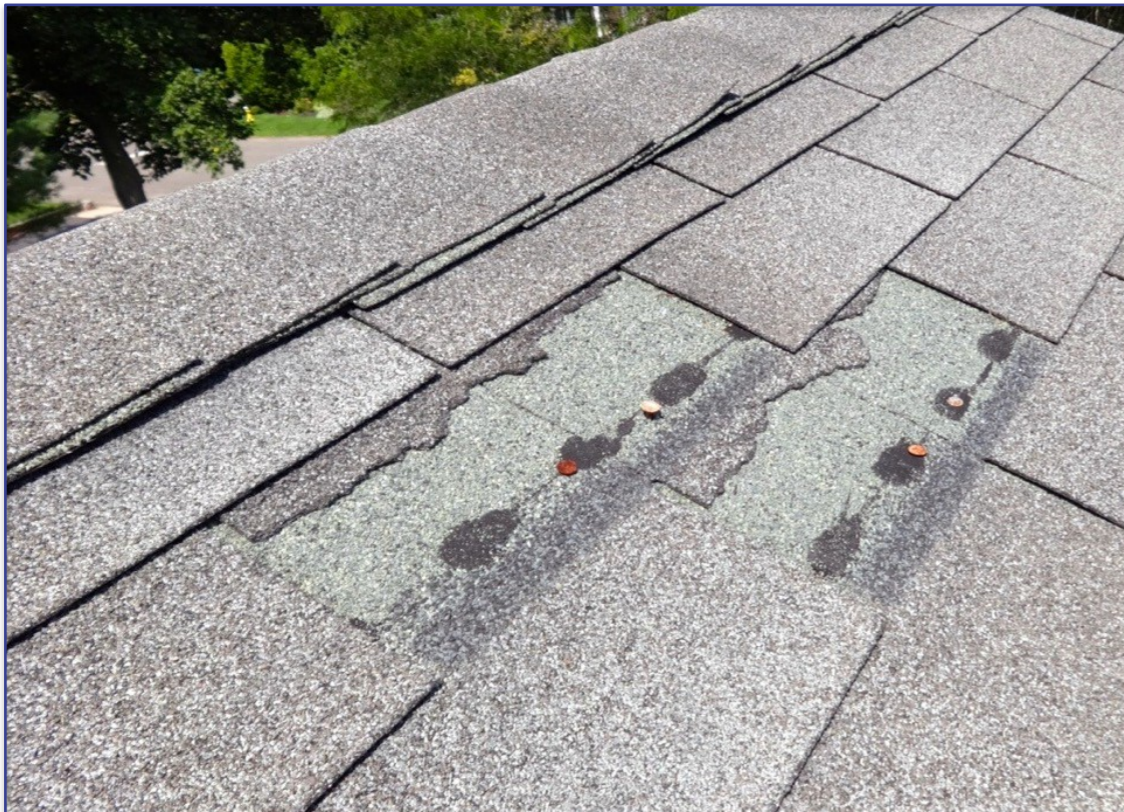
MISSING SHINGLES
