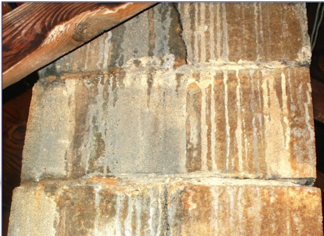
LEAKING CHIMNEY
